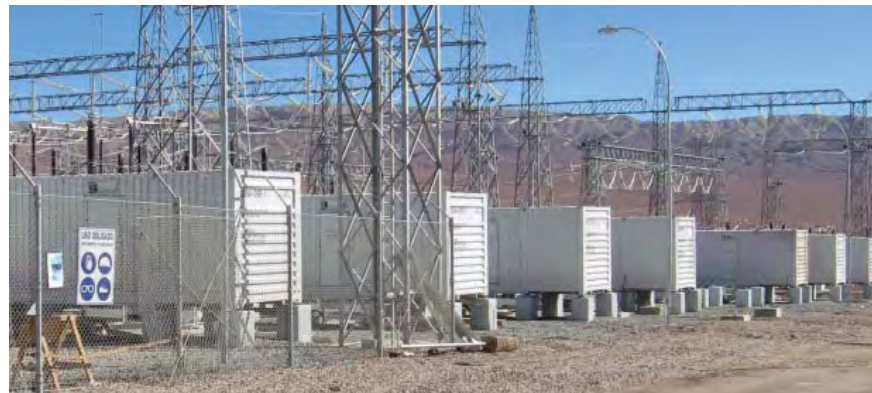
Seven 2 MW A123 modules in operation
