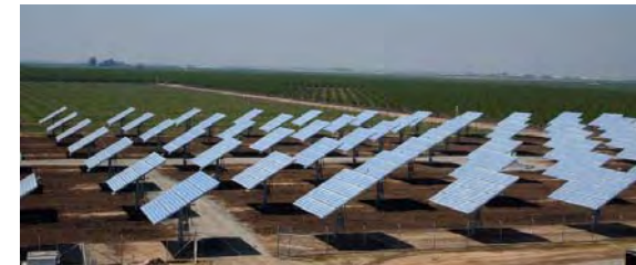
PV collectors on Pedestal Mounts, 1MW system covers 6 acres
