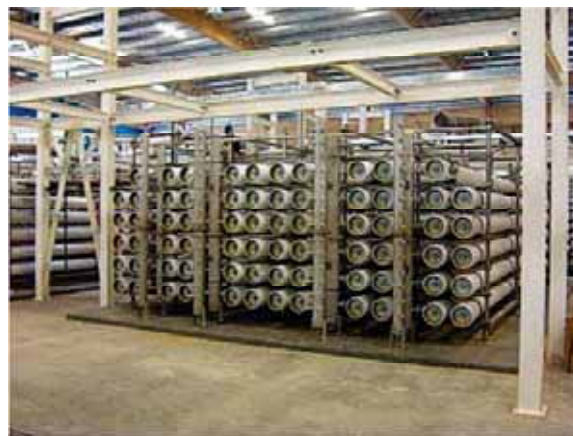
Figure 4-1 Reverse osmosis wastewater treatment Plant, Kuwait
