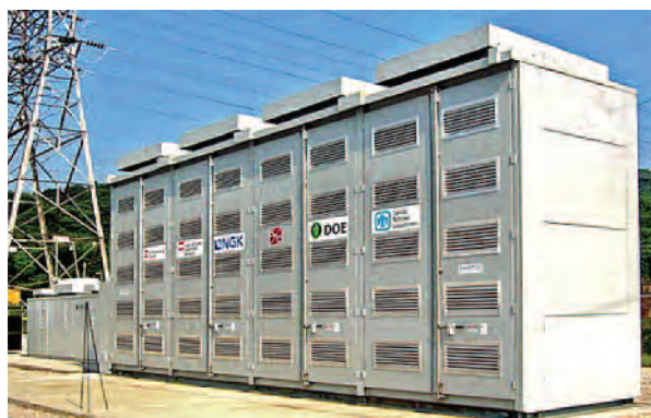
Figure 4.10 Demonstration Unit of Small-Scale Battery Energy Storage
